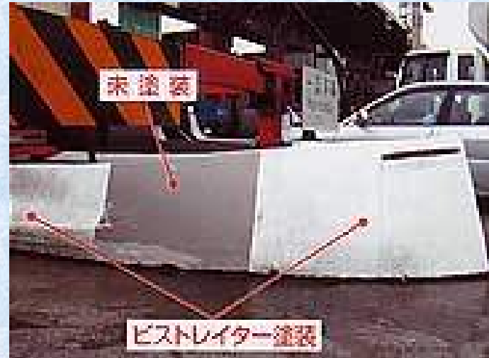
Painting walls in highways
